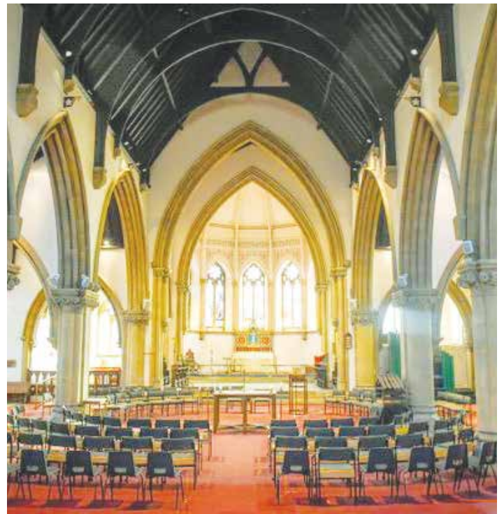
St John's interior, after completion of phase 1 work ("Before", see below)
